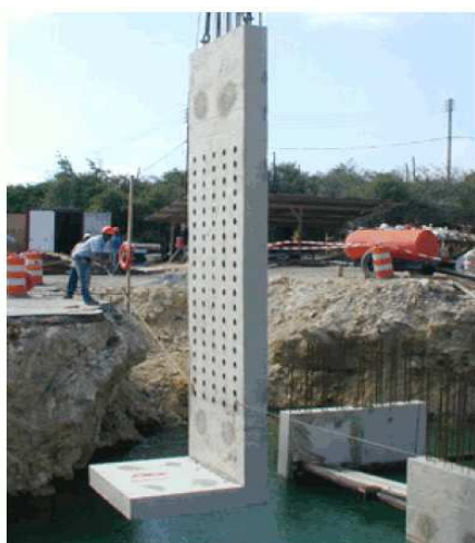
Installation of perforated wall in karst pit
