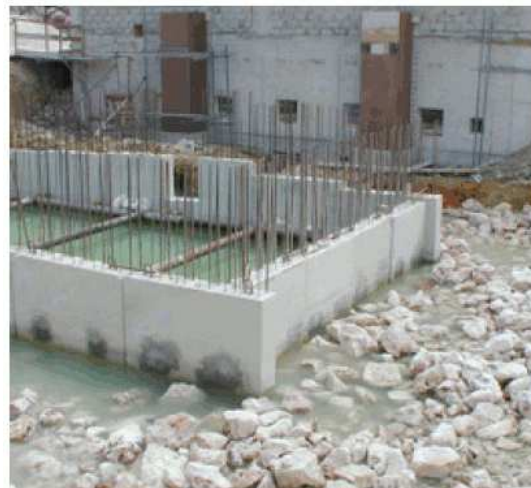
Limestone rocks packed around periphery of karst pit
